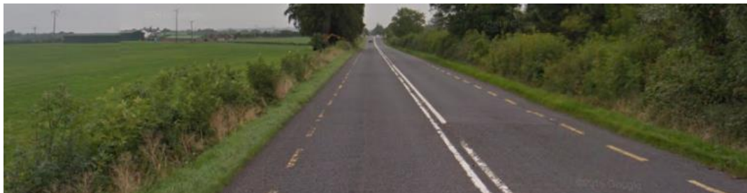
Photo Item No. 14A (Google Street View Image September 2014)
