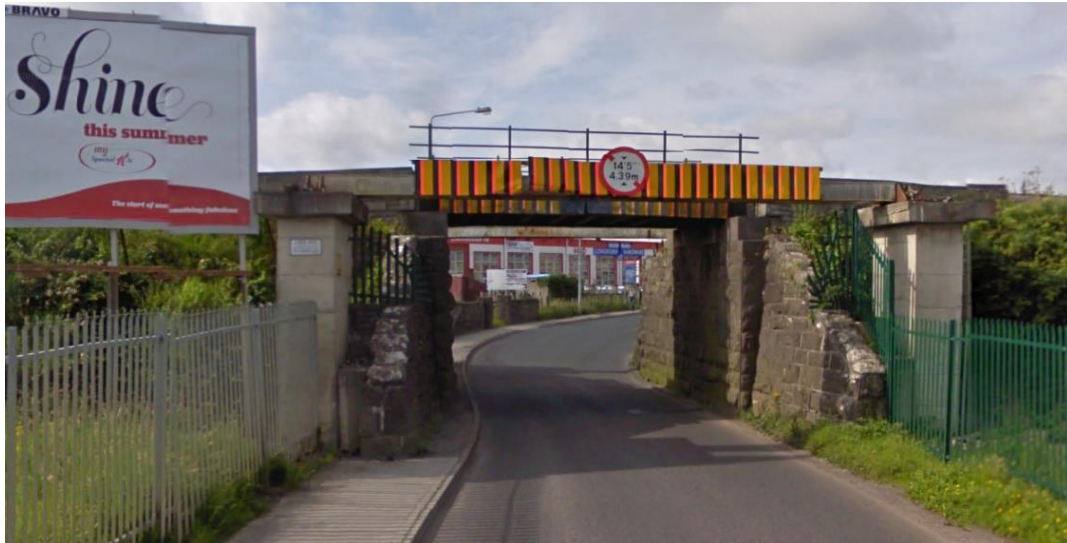
Photo Item No. 27A (Google Street View Image July 2011)
